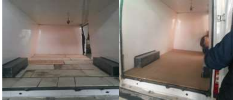
Figure 4. Application of Foam and Particleboard
