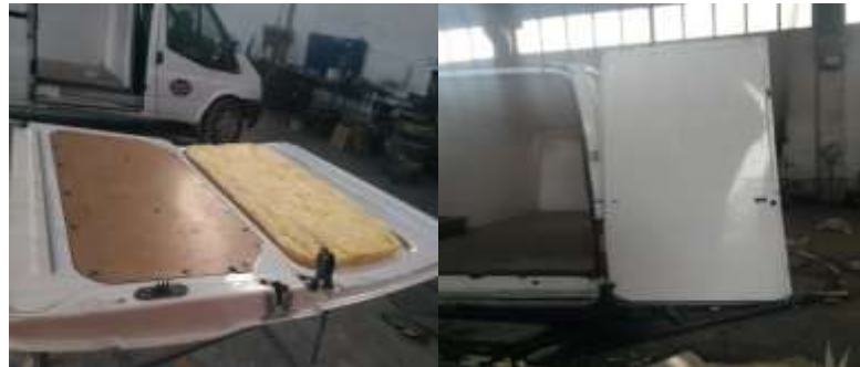
Figure 5. Application of fiberglass and GRP in doors and windows
