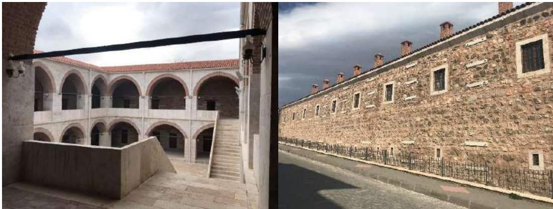
Figure 12. Deveciler Inn Courtyard and Backside View
